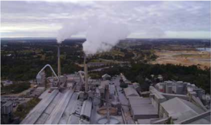
Figure 16. Cockburn Cement Western Australia.
